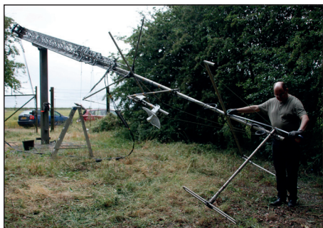
► The East Yorkshire Repeater Group's 20m tower being prepared for a 5m extension to support EY's Alford Slot. The 5GHz grid reflector is used for an Internet feed from G3GJA's QTH.
