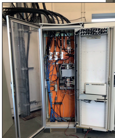
► Receivers, A/V matrix to the left and control PC etc to the right
