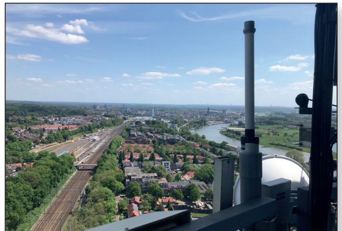
► Facing east towards John Frost Bridge, 3 cm slot aerial to the right, 70 cm aerial bottom and round camera ‘ball’ to the left.
